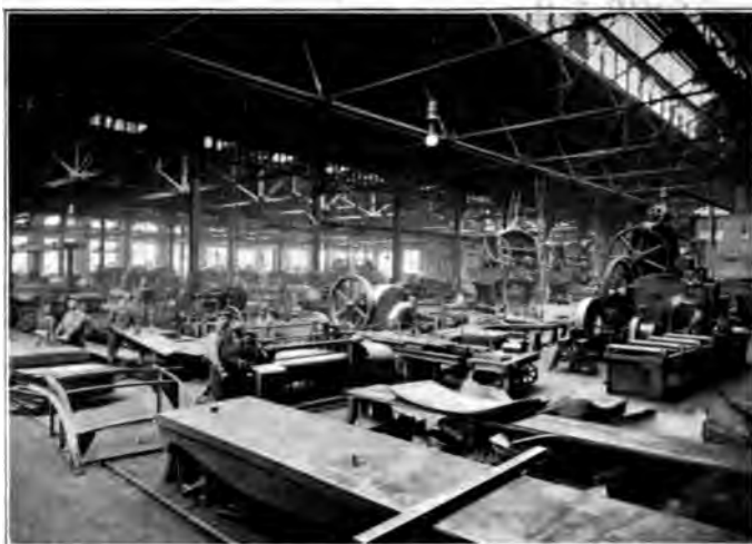
View of machine section. Steel Erecting Shops
